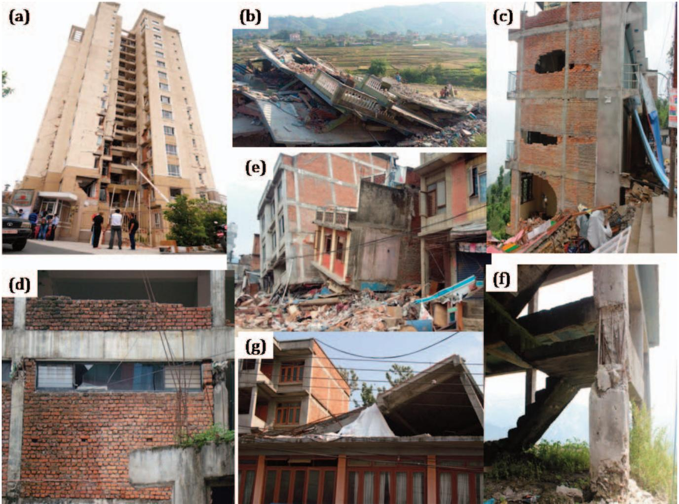
*Fig. 1 - (a) Damaged walls in apartment building (b) Pancake destruction (c) Infill wall damage in residential building (d) Short column (e) Structural pounding (f) Damage in column caused by staircase (g) Collapsed column constructed with welded vertical.*
