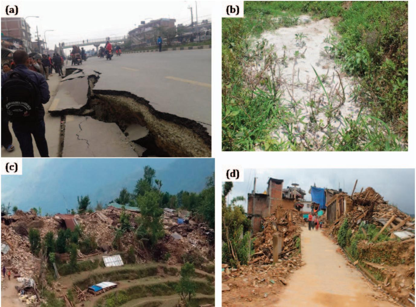
*Fig. 4 - (a) Lateral spreading caused road damage in Kaushaltar; (b) Sand boiling; (c) Completely devastated locality of Mandre (near epicenter); (d) Topographic effect in Chautara (Sindhupalchowk).*
